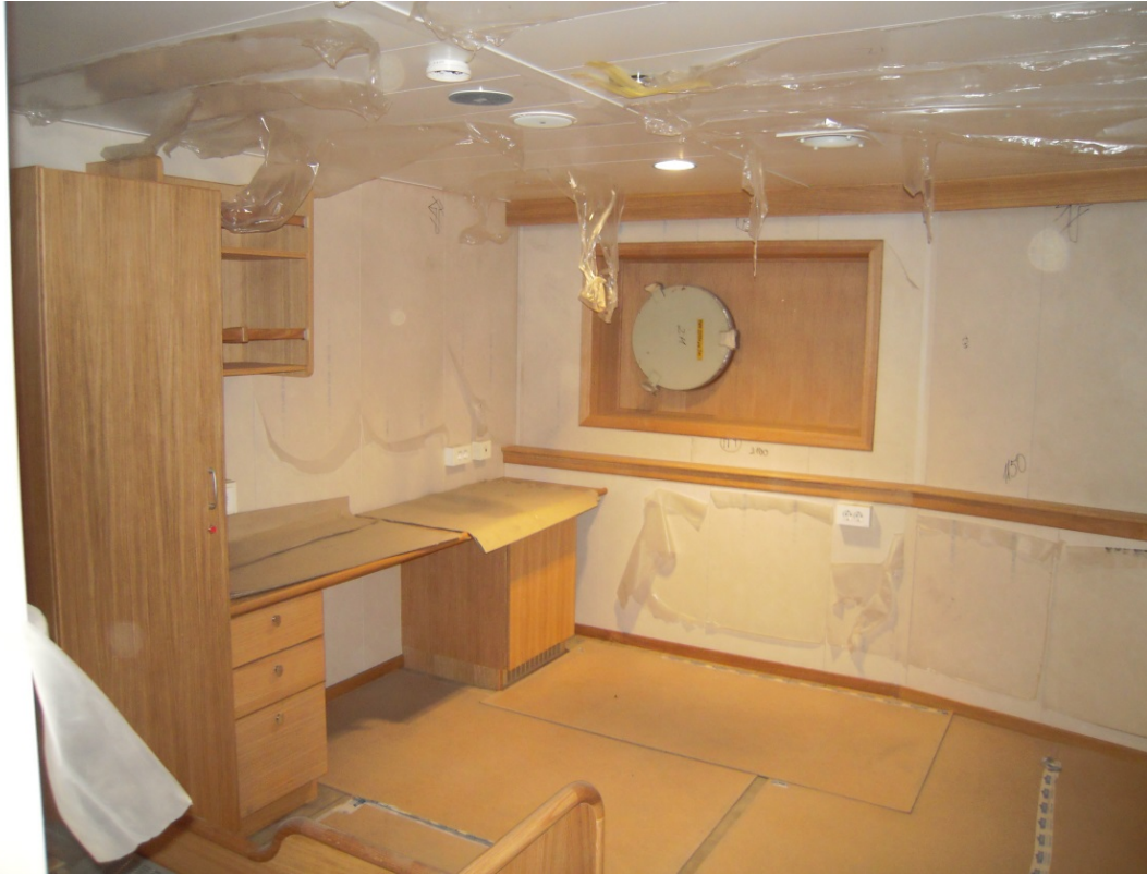
Installation of fixed cabin furniture almost completed
