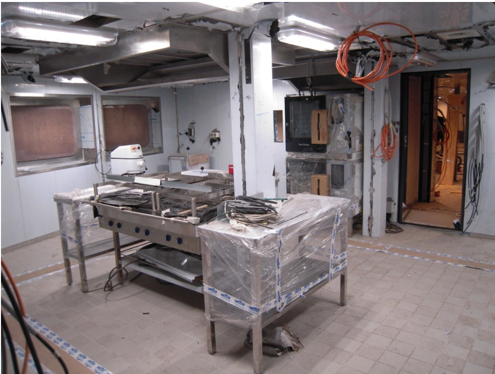
Installation of galley equipment ongoing
