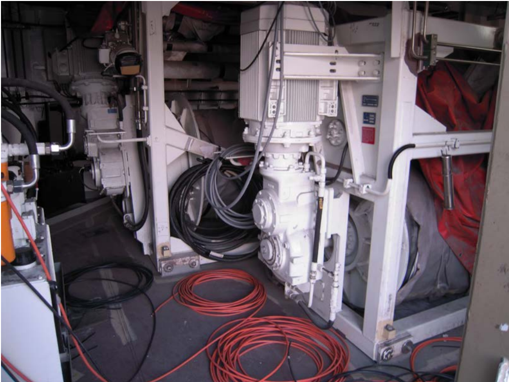
Still some cable pulling and terminations on scientific winches
