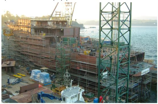
Slipway 30.09 BL 44 (2<sup>nd</sup> dk) installed – (2 more decks to come on top of this!)
